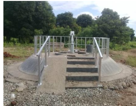
Figure 5: Flood proof borehole construction by SHA and Baseflow in Thyolo
