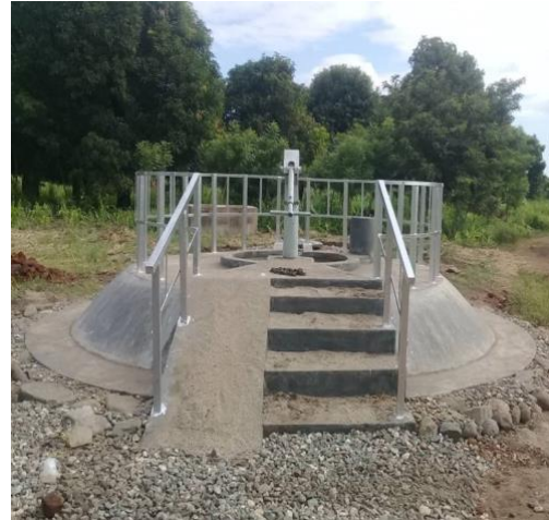
Figure 5: Flood proof borehole (Thyolo)
