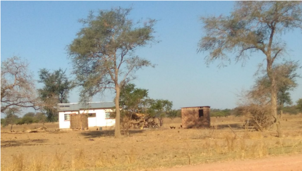
Figure A1.12 - A house for a headman in Itebe
